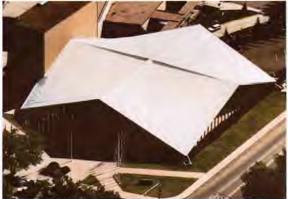
Broadway Convention Center, Colorado Springs, CO. Since 1986, THERMO-SHIELD Roofing System has cured the constant cracking and leaking problem due to lots of movement and thermal shock in this open-span, non-truss roof... supported by cables.
